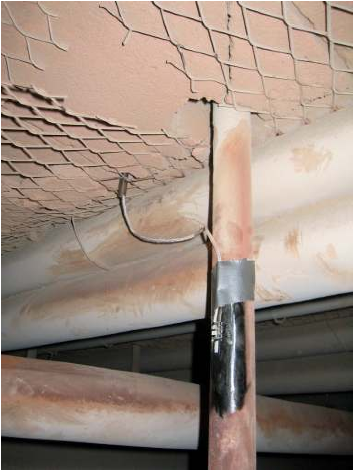
Photo 3, Gage installed on hanger rod
