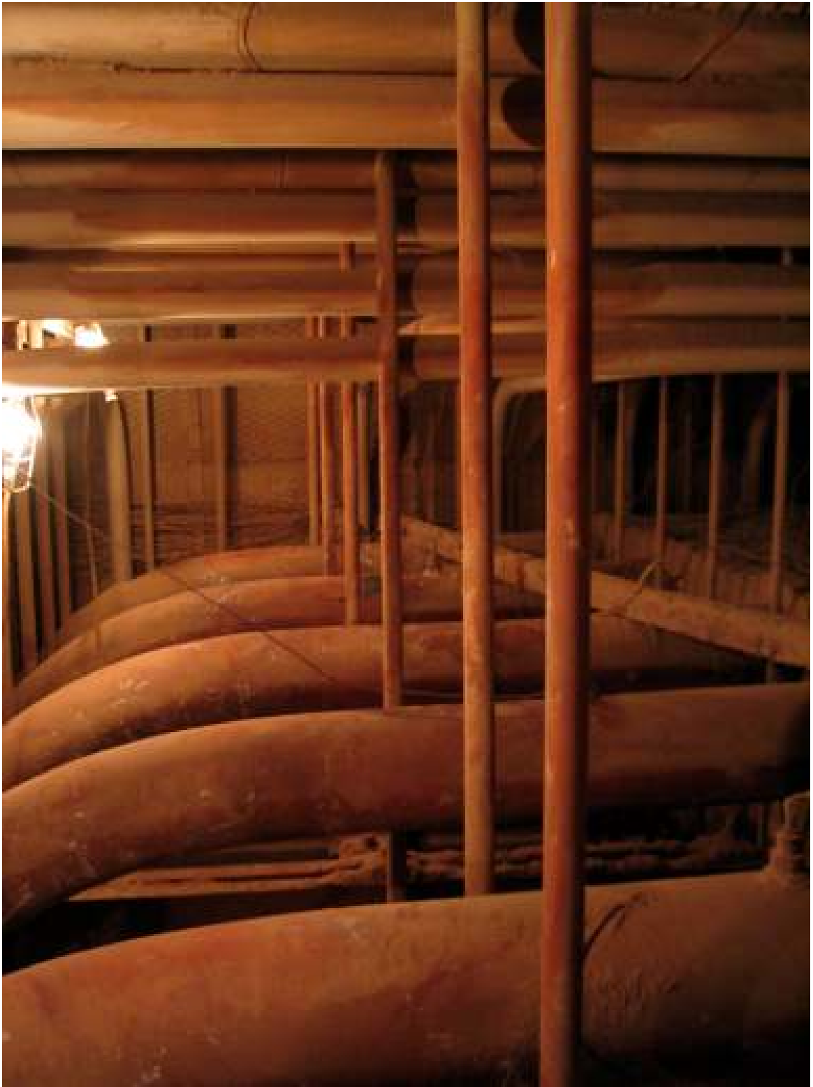
Photo 2, Hanger rods inside penthouse
