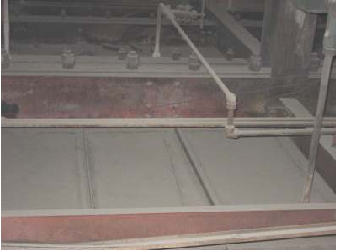
Photo 1, Roof with rod ends visible
