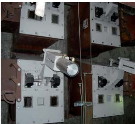
Inboard stacked air ports on the west wall
