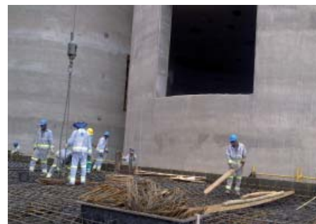
Construction work at the conditioner building
