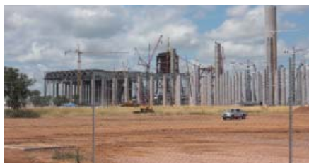
The view from the site offices to the construction site
