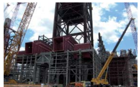
Duct work under construction
